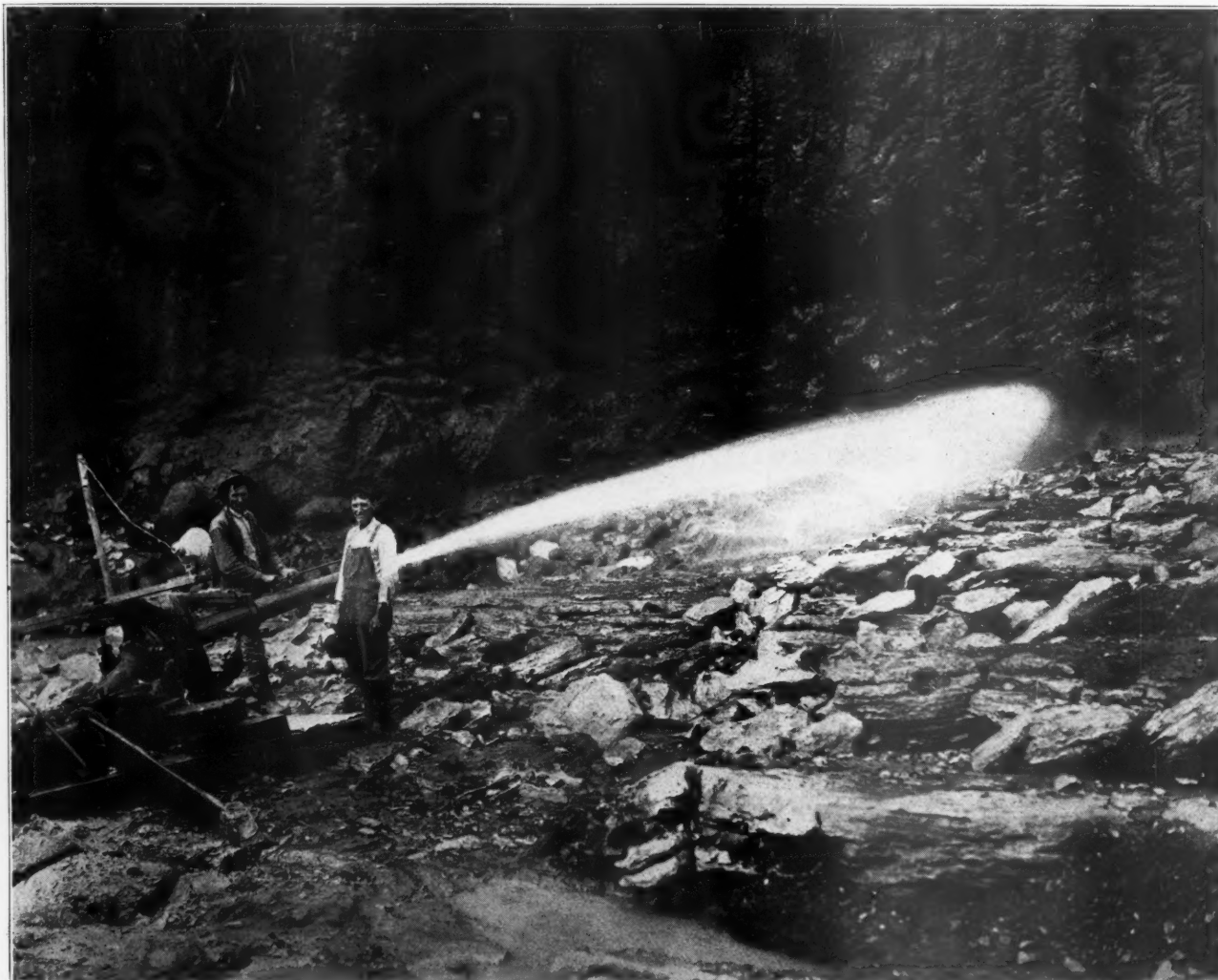
Hydraulic Stripping In a Crushed Stone Quarry
